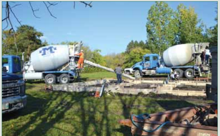
Pouring concrete into the foundation forms.
