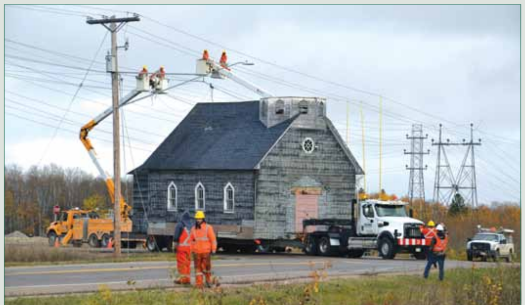
Hydro crews lifting lines at the intersection of PRs 313 and 502.
