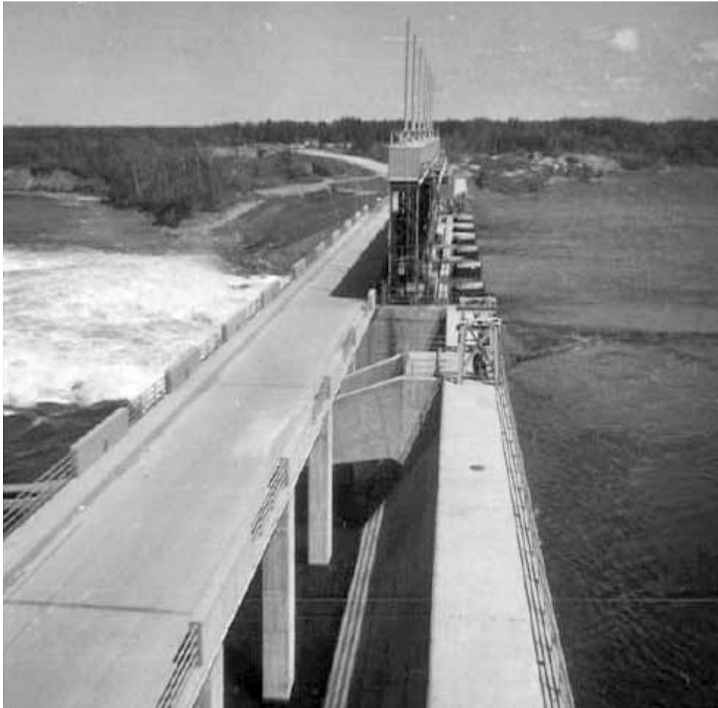
Pine Falls Generating Station with road across, over the Winnipeg River, circa 1952
